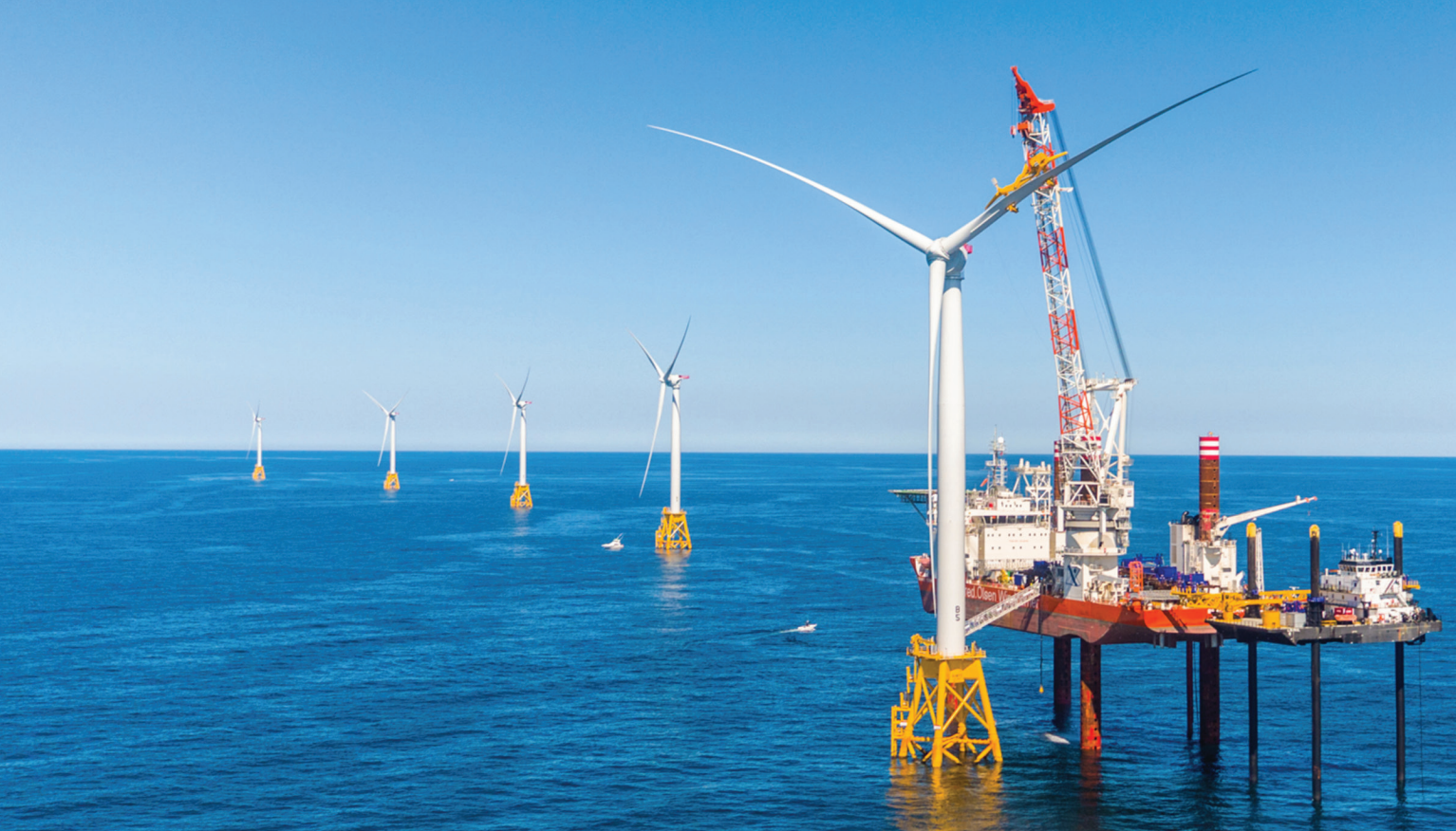
Block Island Wind Farm Construction. Photo: Deepwater Wind
