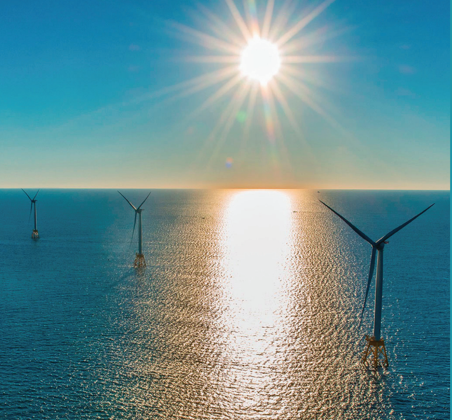
Block Island Wind Farm Sunrise. Photo: Deepwater Wind
